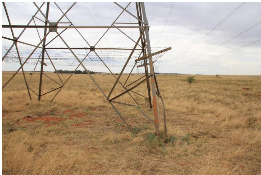
Figure 2: Deformed truss and bracing members
