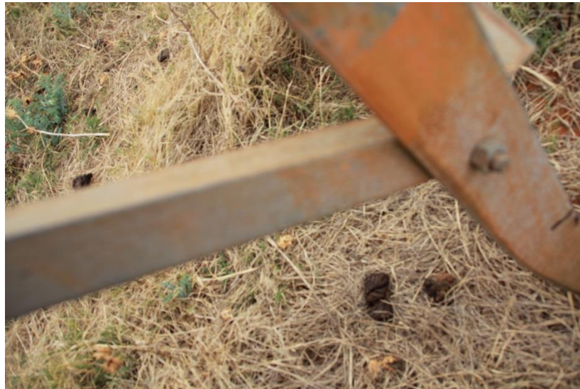
Figure 1: Deformed main member of the leg
